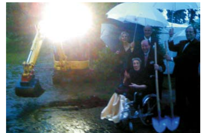
Ground breaking for the new John E. Palmer '64 Theater
